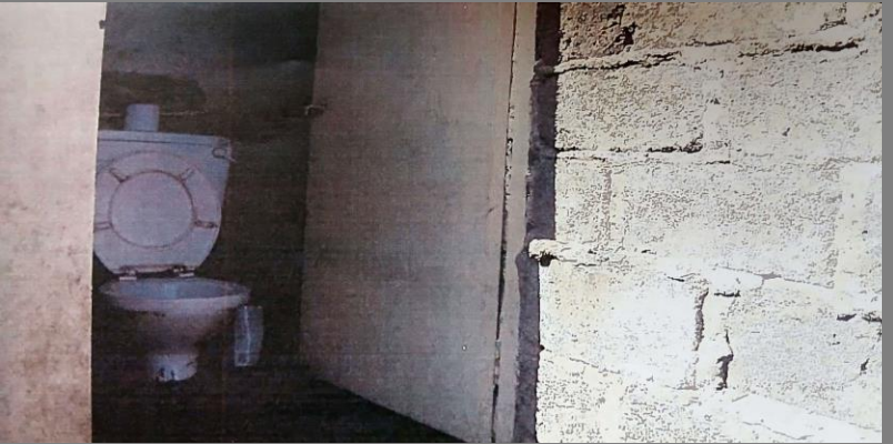
The only outside toilet.
