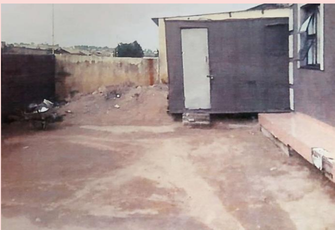
Construction of the new home.
